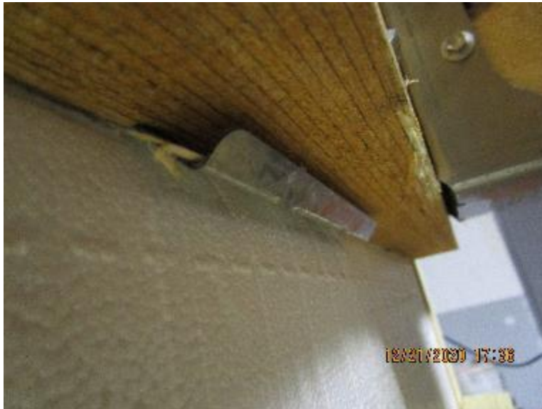
Photo No. 5 Typical ICF Wood Ledger Failure
