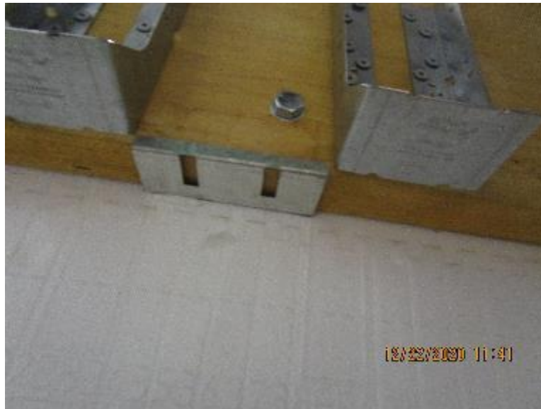
Photo No. 2 ICF Wood Ledger with Joist Hangers Attached
