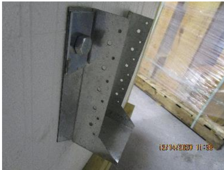
Photo No. 1 ICF Joist Hanger
