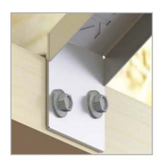
Install bottom brace to I-joist as shown (3 screws each leg).
