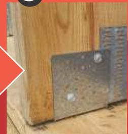
Screw fix roof truss/rafter each side to BHB anchor using
