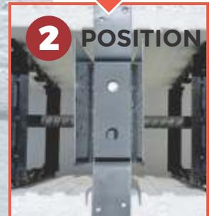
Position BHBCON at truss/rafter mark
