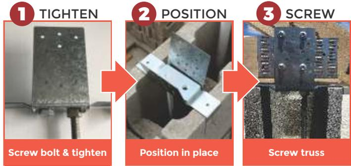
1. Screw J-Bolt and tighten nut to BHBCON prior to concrete pour
